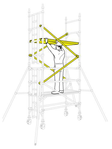
Climb up the inside of the tower and from the protected position of the trapdoor, fit guardrails to the 7th and 8th rungs, (in that order), on both sides of the tower.
