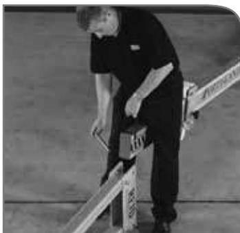
Offer the beam to the rear bolt-hole on the cheek-plate (Bolt 1) and insert a bolt. Put on plain & spring washers and nut finger tight.
