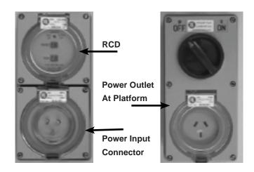
Figure 2.13 - RCD/ELCB AC Outlet
