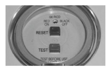
Figure 5.2 - RCD / ELCB Outlet
