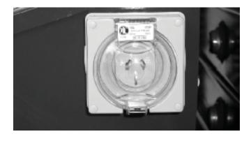
Figure 11.7 - Mains Power Connection For Charger
