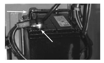
Figure 7.12 - Battery Terminals
